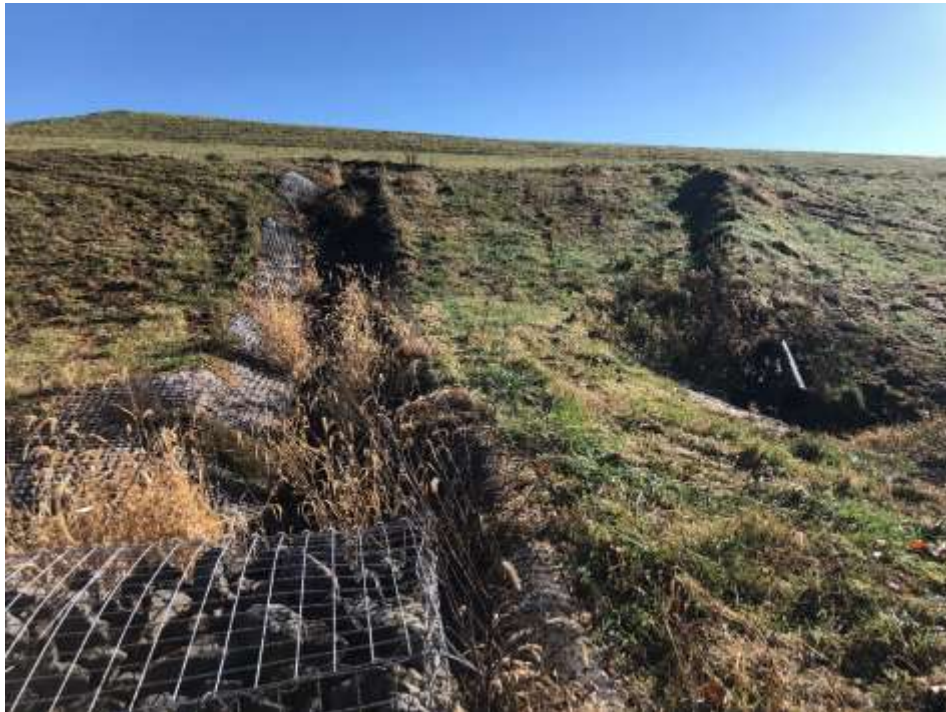
Photograph 28: Non-contact stormwater downchute is clear of obstructions. Gabion energy dissipator is installed at the junction with the stormwater perimeter ditch.
