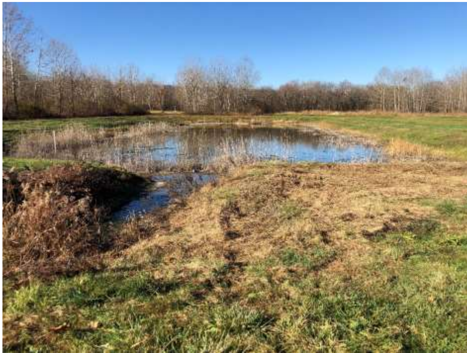
Photograph 33: Leachate (contact water) Pond. No evidence of animal burrows or liner damage.
