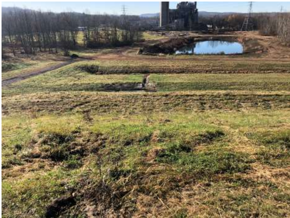
Photograph 12: Stage 4 south slope is well vegetated and mowed annually. No evidence of animal burrows, erosion, or stability issues.
