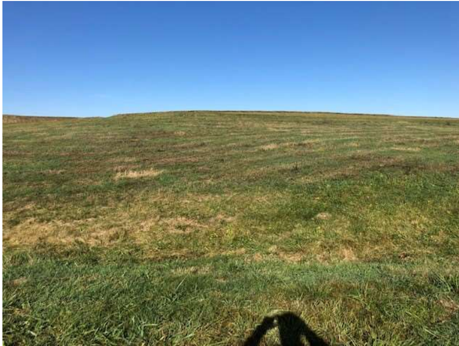
Photograph 45: Southeast corner final cover lower slope is well vegetated and mowed annually. No evidence of animal burrows, erosion, or stability issues.
