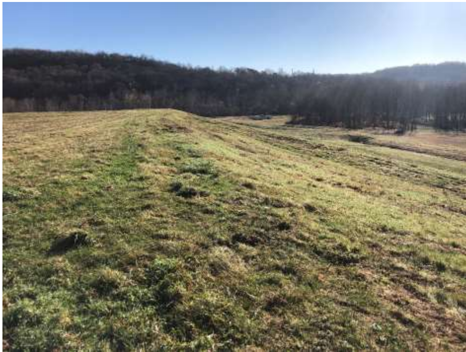
Photograph 9: Stage 4 south slope is well vegetated and mowed annually. No evidence of animal burrows, erosion, or stability issues.
