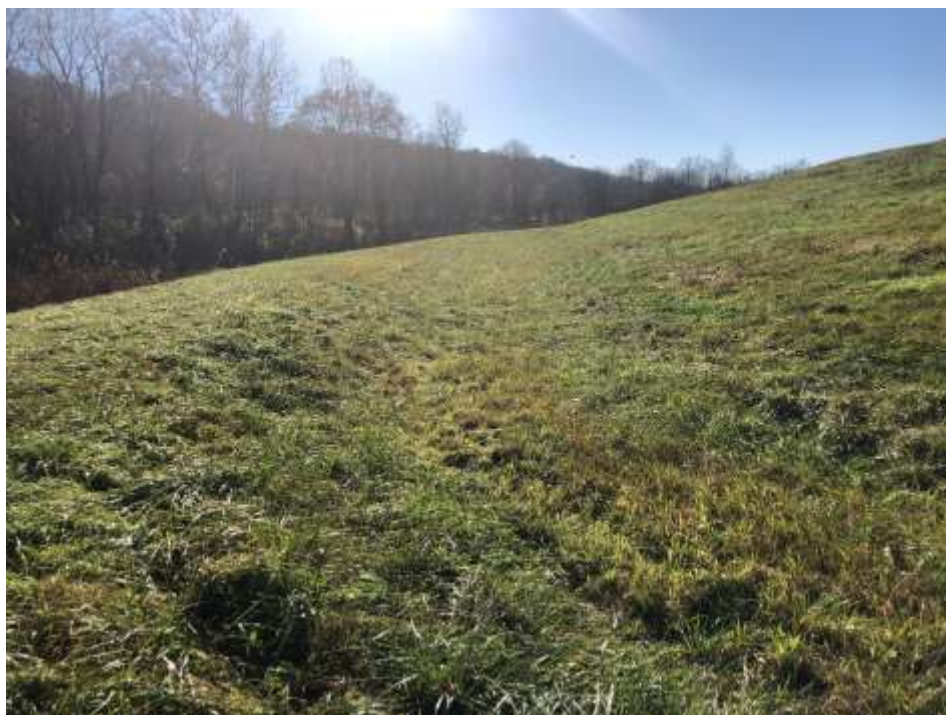
Photograph 38: East non-contact stormwater channel is clear of obstructions. East final cover lower slope is well vegetated and mowed annually. No evidence of animal burrows, erosion, or stability issues.
