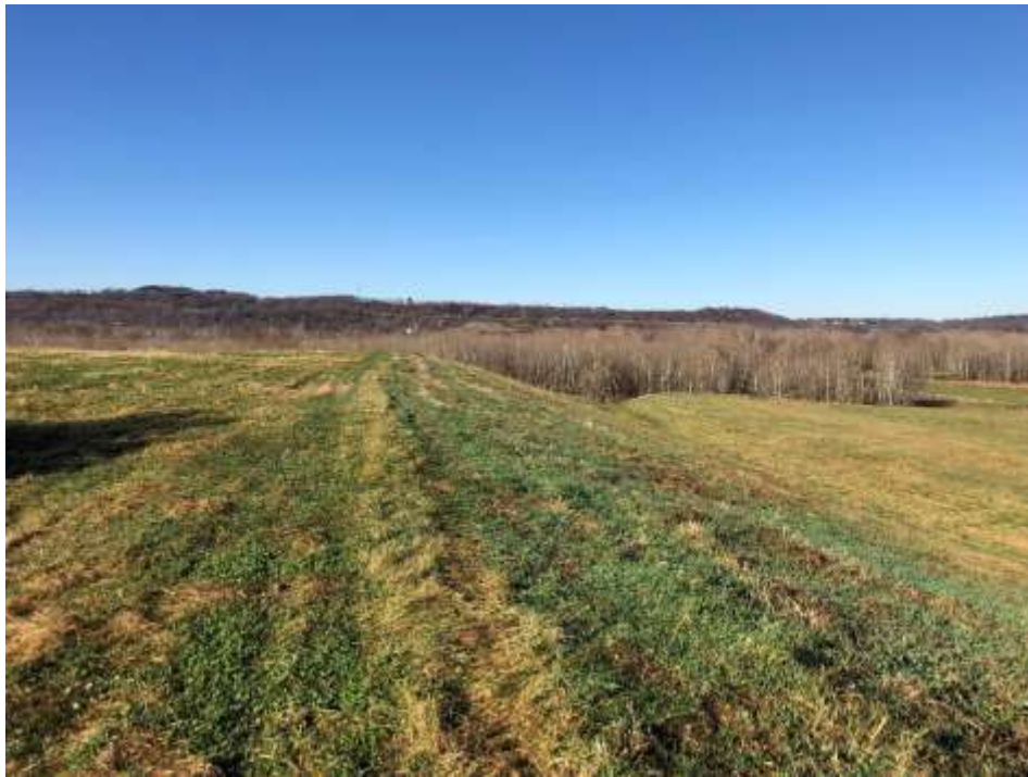
Photograph 5: Stage 4 north slope is well vegetated and mowed annually. No evidence of animal burrows, erosion, or stability issues.
