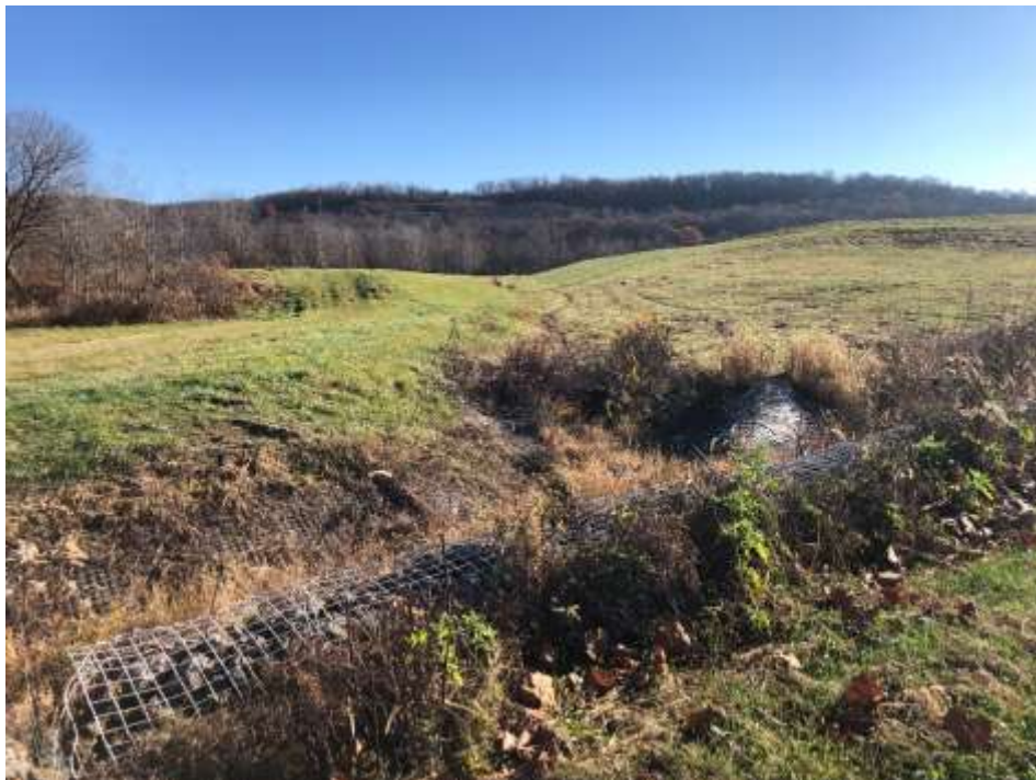
Photograph 32: North non-contact stormwater channel is clear of obstructions. North final cover lower slope is well vegetated and mowed annually. No evidence of animal burrows, erosion, or stability issues.
