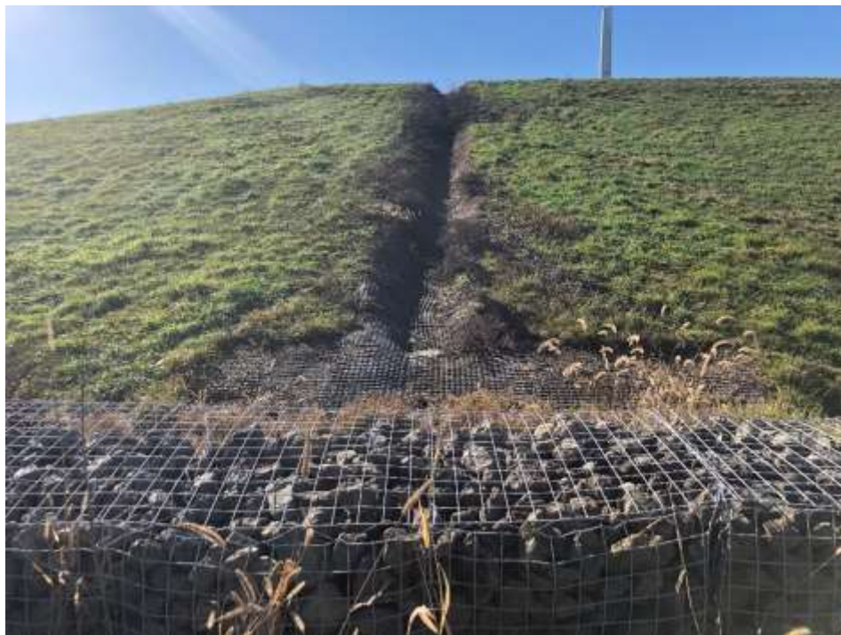
Photograph 37: Non-contact stormwater downchute is clear of obstructions. Gabion energy dissipator is installed at the junction with the stormwater (non-contact water) perimeter ditch.
