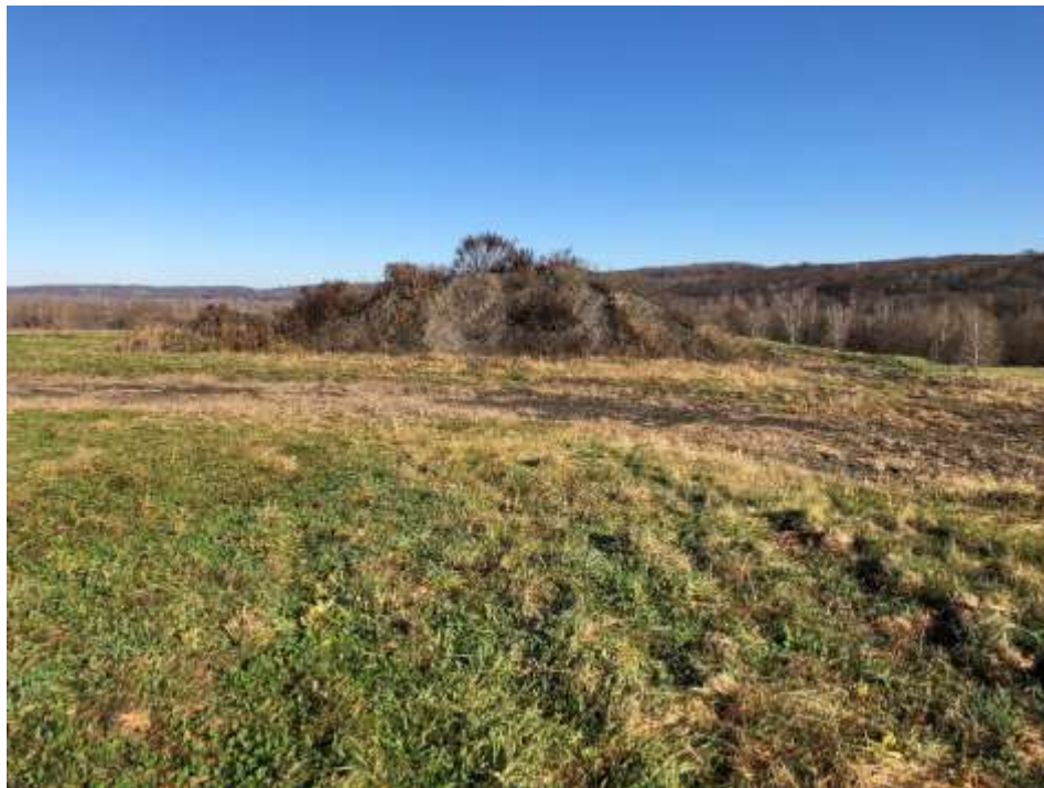
Photograph 17: Intermediate cover in active area is well vegetated and mowed annually. Bottom ash storage pile.
