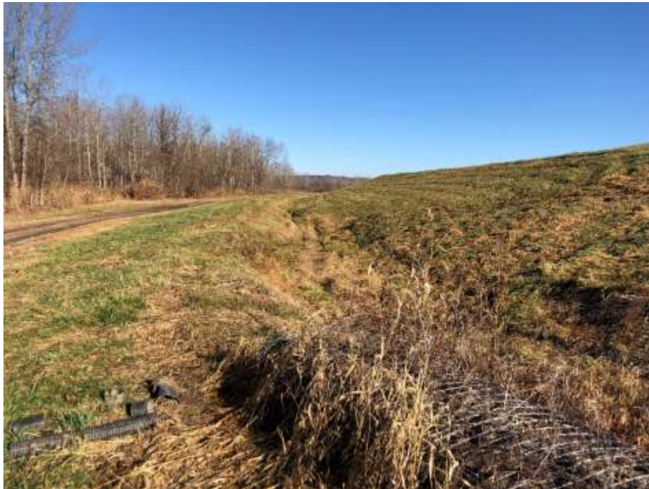
Photograph 26: West non-contact stormwater channel is clear of obstructions. West final cover lower slope is well vegetated and mowed annually. No evidence of animal burrows, erosion, or stability issues.
