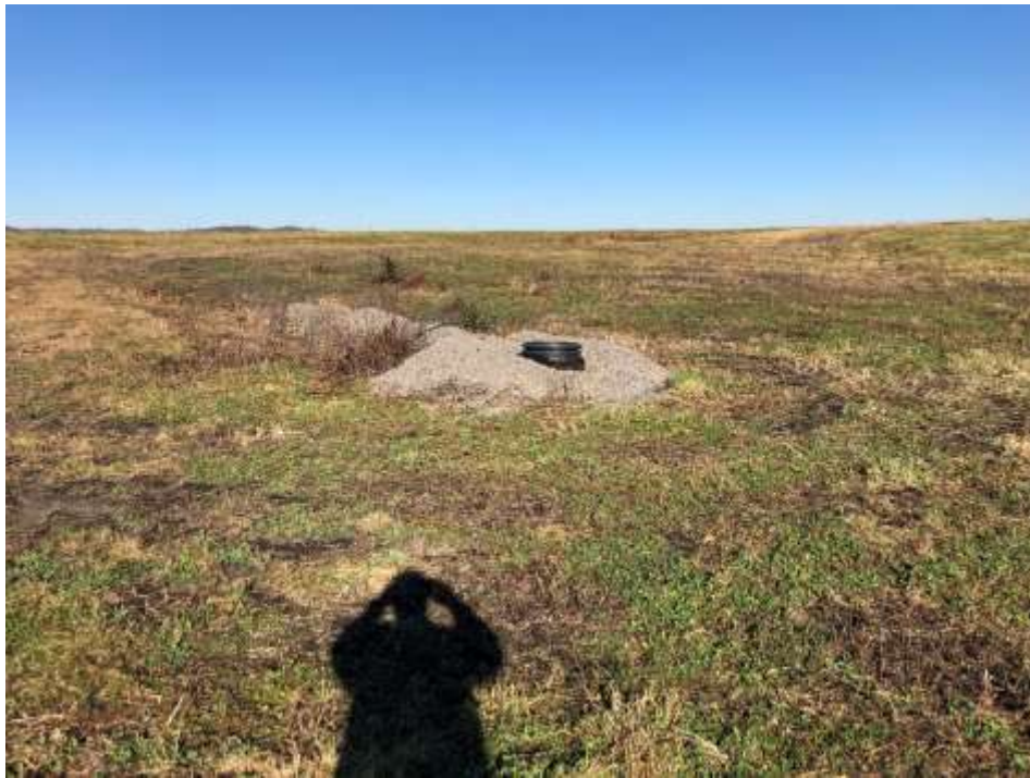
Photograph 15: Contact water collection riser in active area.
