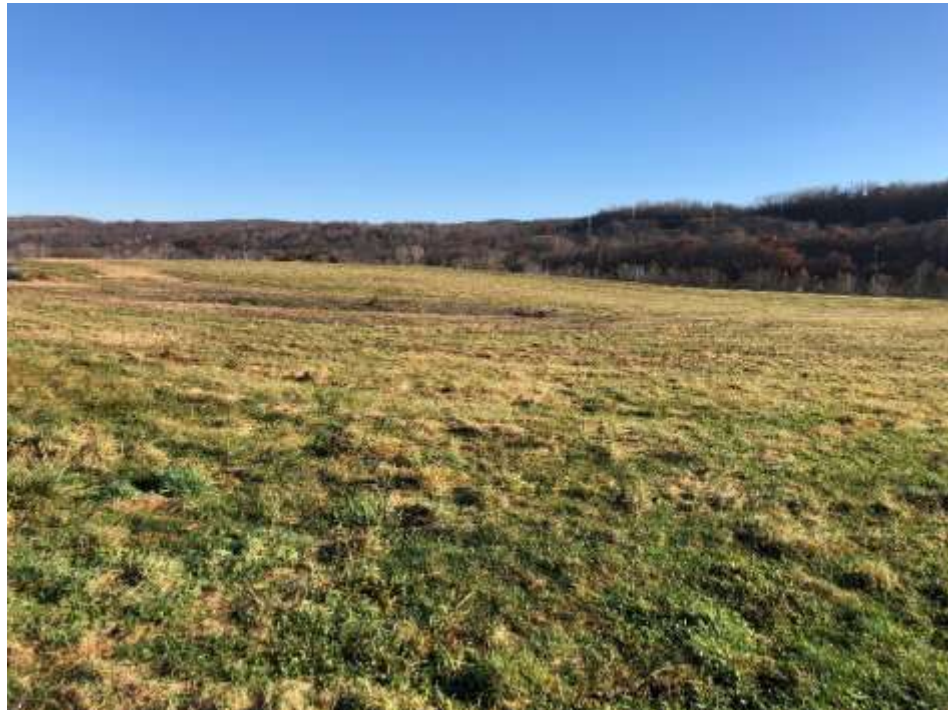
Photograph 10: Intermediate cover in active area is well vegetated and mowed annually.
