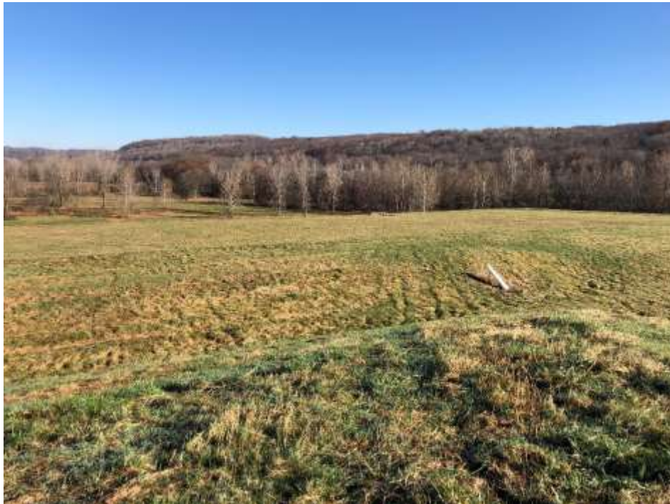
Photograph 2: Stage 5 final cover is well vegetated and mowed annually. No evidence of animal burrows, erosion, or stability issues.
