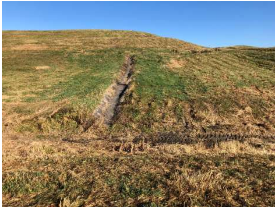
Photograph 24: Non-contact stormwater downchute is clear of obstructions.
